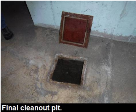
Final cleanout pit.
